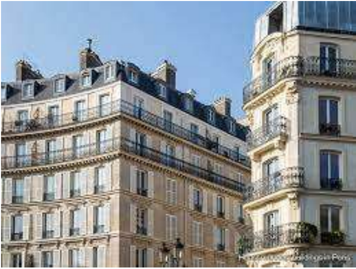
Style architectural haussmanien
